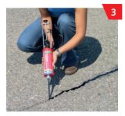
Quickly fill the contents of the cartridge into the cleaned joint, using up the mixture completely as the curing process starts quickly.
