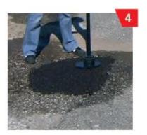
Compact well using a tamper. For larger areas, a roller or vibratory plate compactor is recommended.
