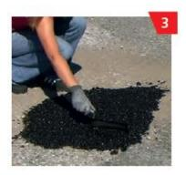
Use a rake or a trowel to lay the repair asphalt slightly above the surface.
