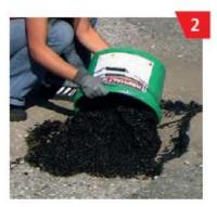
$\mbox{Mix}$  REPHALT® homogeneously with approx. 2  $\mbox{M}\%$  water and then apply to the damaged area.
