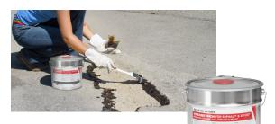
To improve adhesion between the existing asphalt or concrete surface and the **REPHALT**<sup>®</sup> or **REFUG**<sup>®</sup>.
