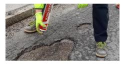
In a practical 750 ml spray can to improve adhesion between the existing asphalt or concrete surface and the **REPHALT**<sup>®</sup> or **REFUG**<sup>®</sup>.
