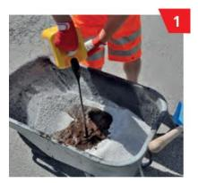
The sand is places in a mixing container and then the bitumen emulsion is added.
