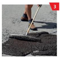
Spread quickly using a rubber spreader or towel and level out.
