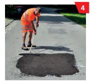
Depending on the weather and installation thickness, the laid mix can be driven on after approx. 30 minutes.
