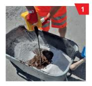
The sand is placed in a mixing container and then the bitumen emulsion is added.
