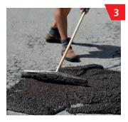
Spread quickly using a rubber spreader or trowel and level out.
