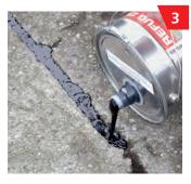
Process the finished mixture quickly, as the curing process starts to happen quickly.
