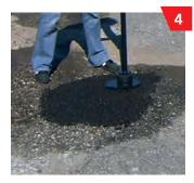
Compact well using a tamper\*. For larger areas, a roller or vibratory plate compactor is recommended.
