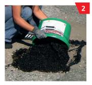
Mix **REPHALT**<sup>®</sup> homogeneously with approx. 2 M% water and then apply to the damaged area.
