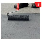
... and roll off in pore-filling strips using a sealing roller\*.
