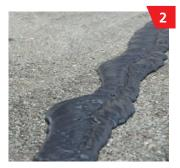
Mask the surface at the edges using a suitable adhesive tape\* and then pour **STRADAFIX®** onto the underlay in portions.
