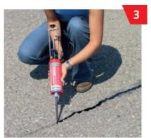
Quickly fill the contents of the cartridge into the cleaned joint, using up the mixture completely as the curing process starts quickly.
