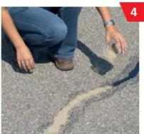
The filled joint can be removed using a spatula and sprinkled with chippings or sand.
