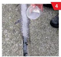
The filled joint can be sprinkled with chippings or sand.
