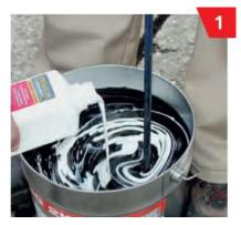
Stir component A thoroughly using a suitable stirring device and then stir in component B.
