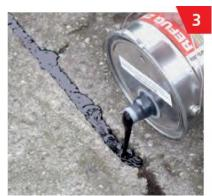
Process the finished mixture quickly, as the curing process starts to happen quickly.
