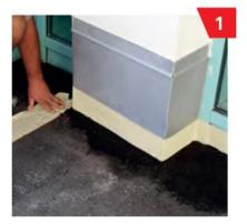
Thoroughly clean the surface and carefully mask the edges with a suitable adhesive tape. Lay the plastic fabric inlay and fix it with RESIST FibreGlue.
