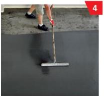
Then spread with a suitable rubber slider and thinly peel off – pay attention to the minimum quantity of 2 kg/m<sup>2</sup>.
