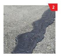
Mask the surface at the edges using a suitable adhesive tape and then pour STRADAFIX $^{\circledR}$  onto the underlay in portions.
