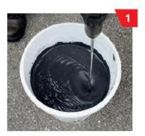
Mix STRADAFIX® homogeneously using a suitable stirring device.
